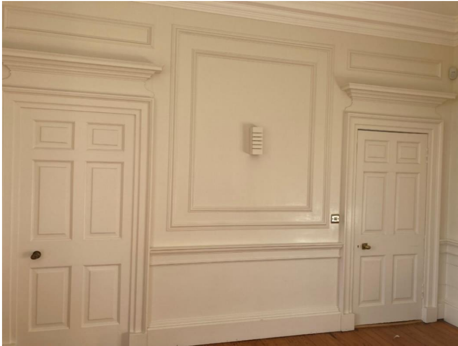
Figure 35 Later 18th Century panelling restored in the Dining Room
