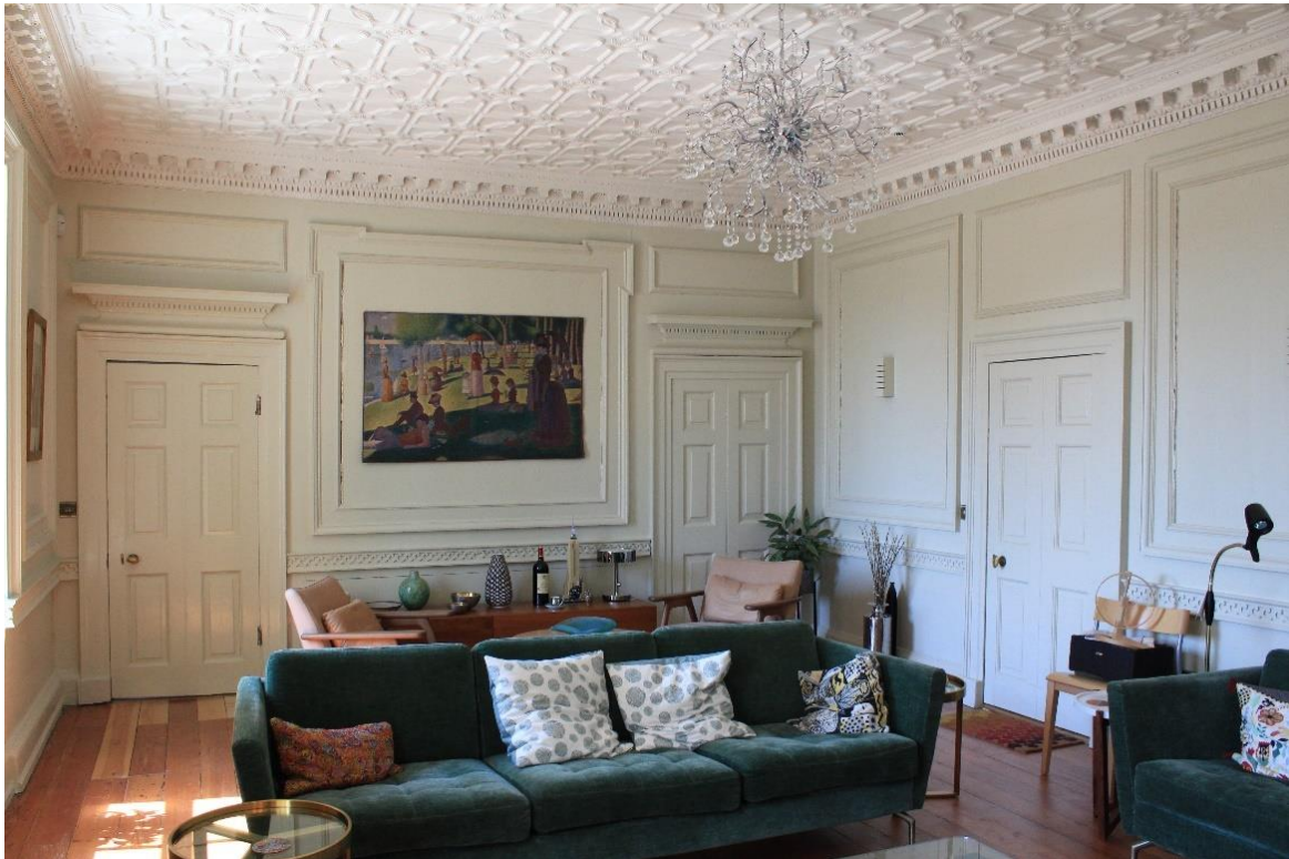
Figure 34 Living Room with restored 18th Century Panelling and 19th Century Lincrusta ceiling.
