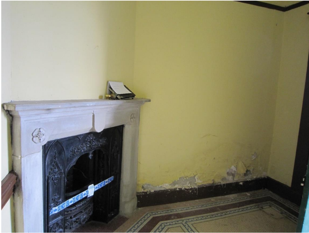
Figure 40 Typical damp problems to the ground floor
