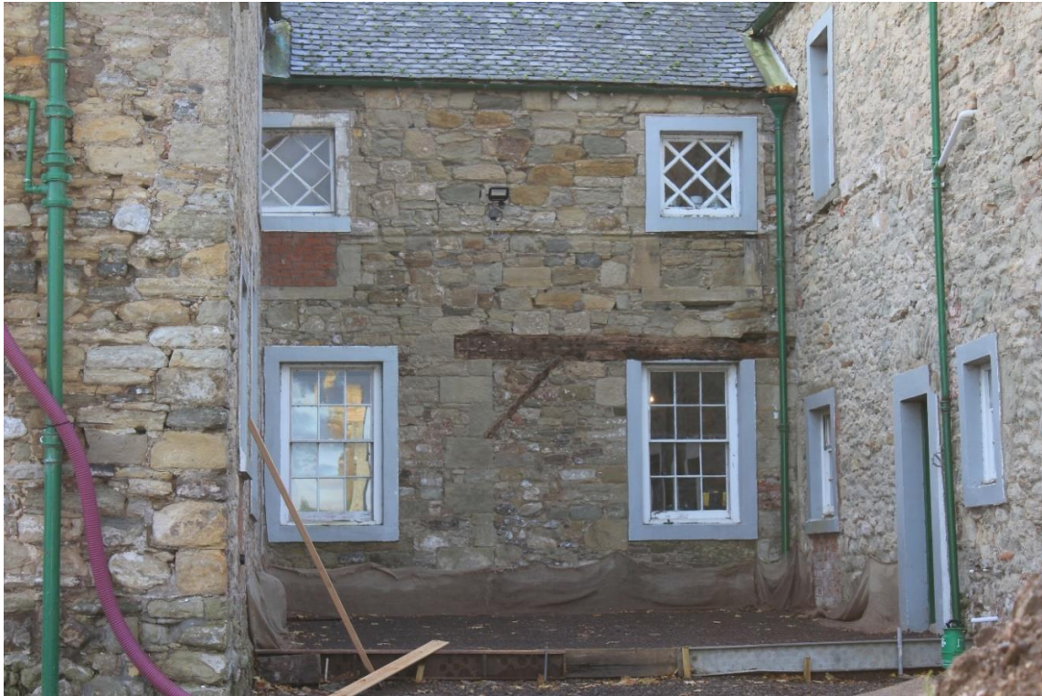
Figure 21 Location of former opening into corridor
