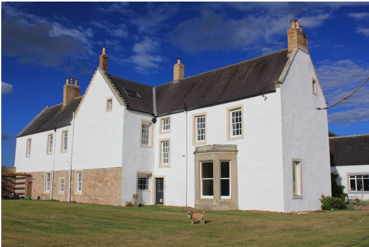
Figure 51 The restored east elevation
