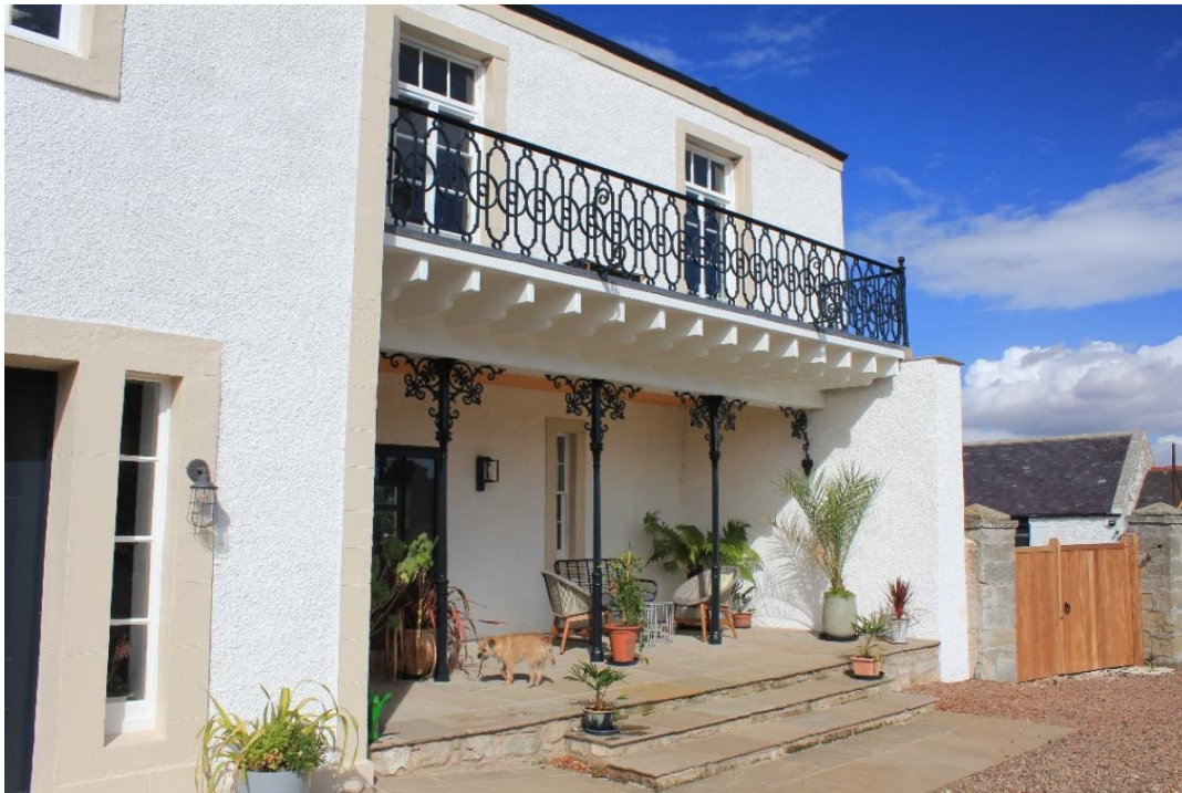
Figure 47 The restored balcony
