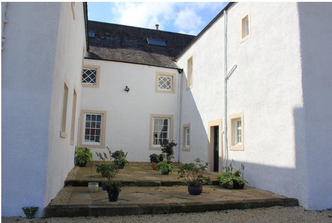
Figure 49 The north courtyard repaved and restored.
