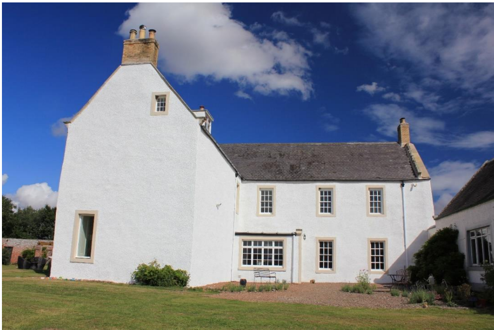
Figure 43 The house re-rendered and painted
