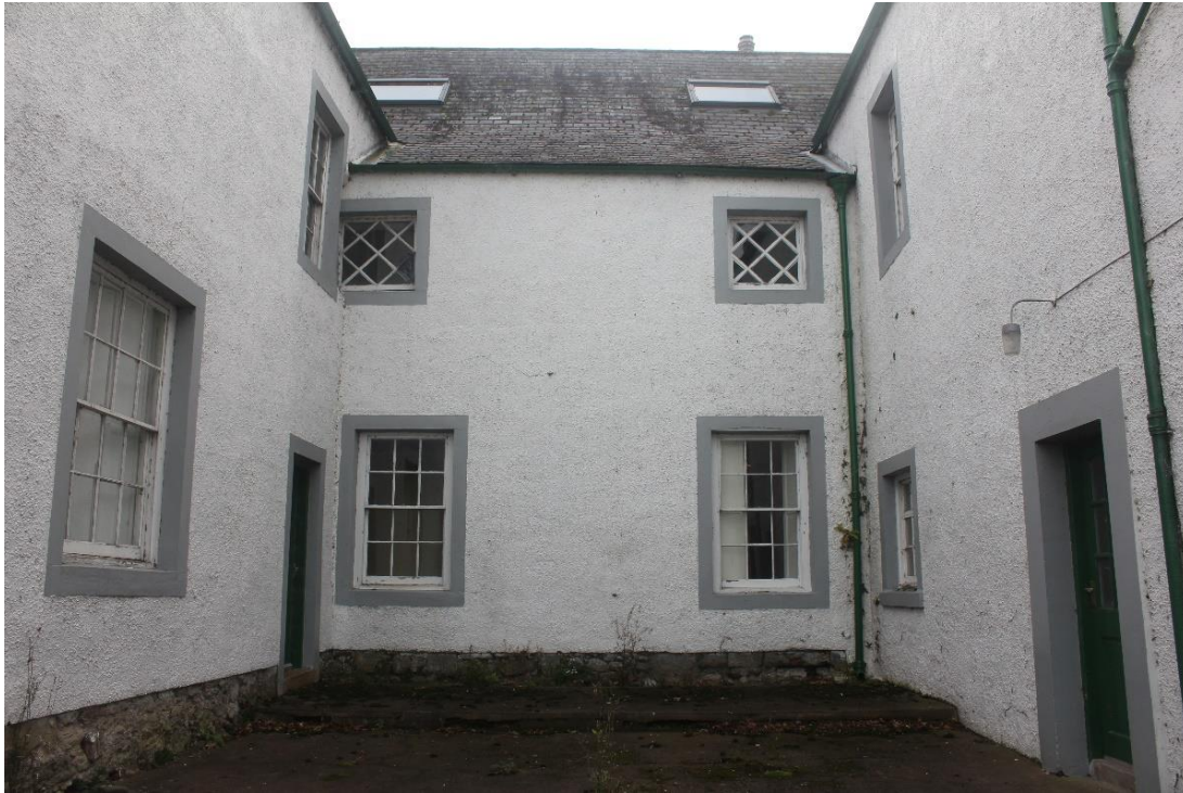
Figure 48 The north courtyard before restoration
