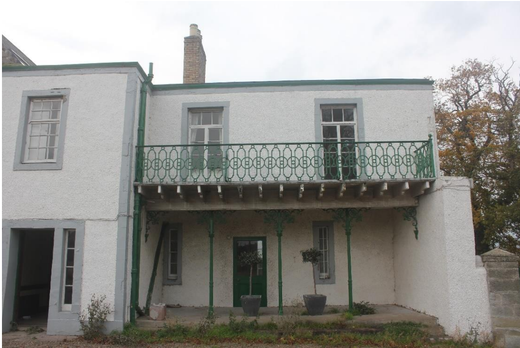
Figure 46 Existing condition of the Victorian ironwork
