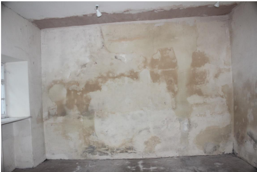
Figure 41 Extreme damp conditions in the ground floor
