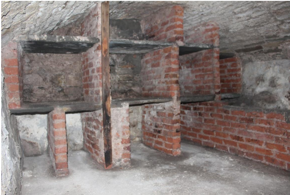
Figure 25 The cellar under the Northeast wing
