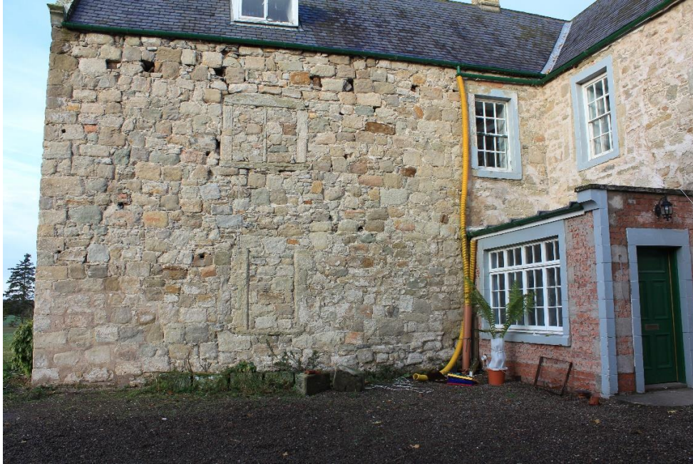
Figure 23 Earlier window pattern visible in the stonework
