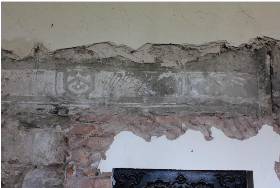
Figure 17 Forster Coat of Arms revealed on chimney breast when plaster removed in reception room
