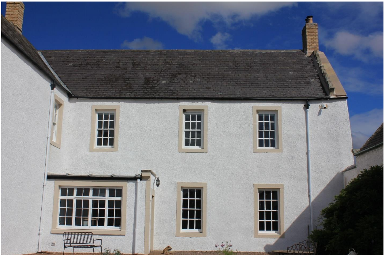
Figure 33 Georgian Windows inserted into 16th Century fabric
