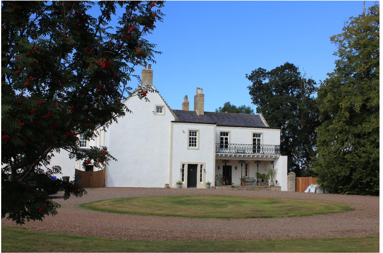
Figure 52 The restored west elevation
