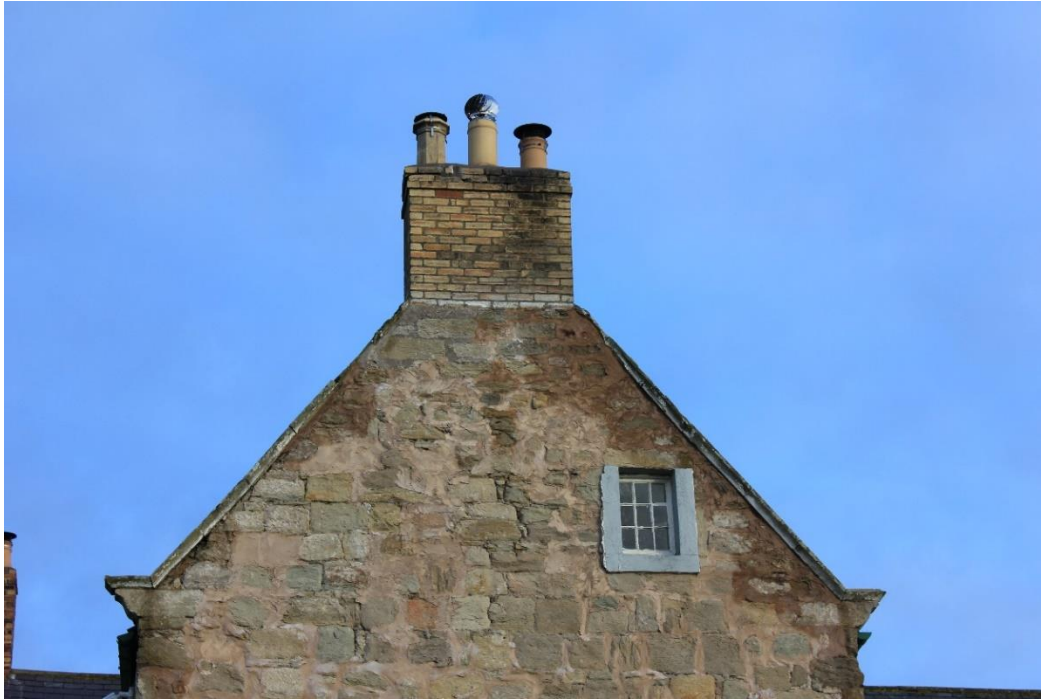
Figure 42 Vertical cracks discovered in the gable walls were stitched with ss rods
