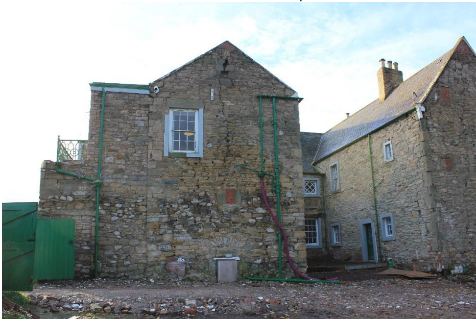
Figure 24 Clay built gable visible on ground floor of northeast wing
